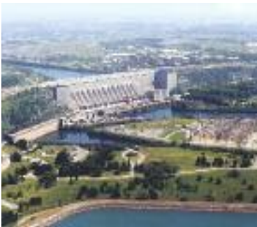
Sir Adam Beck Hydroelectric Project
