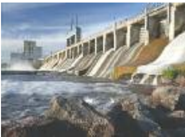
Seven Sisters Generating Station, Manitoba
