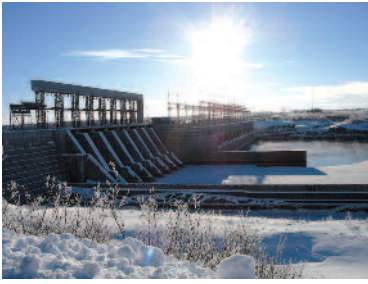
La Grande 1 Power Station of the James Bay Complex
