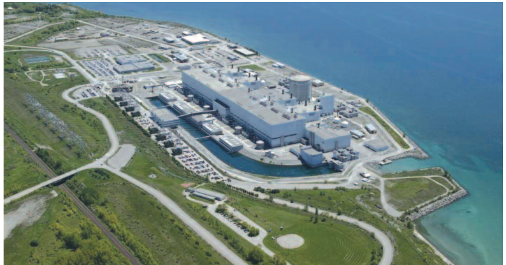
Four Reactor CANDU Darlington Plant, Ontario Power Generation
