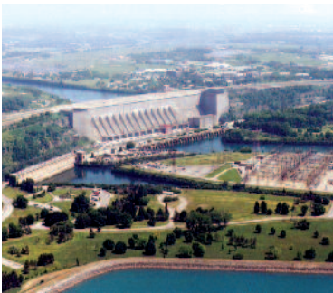
Sir Adam Beck Hydroelectric Project
