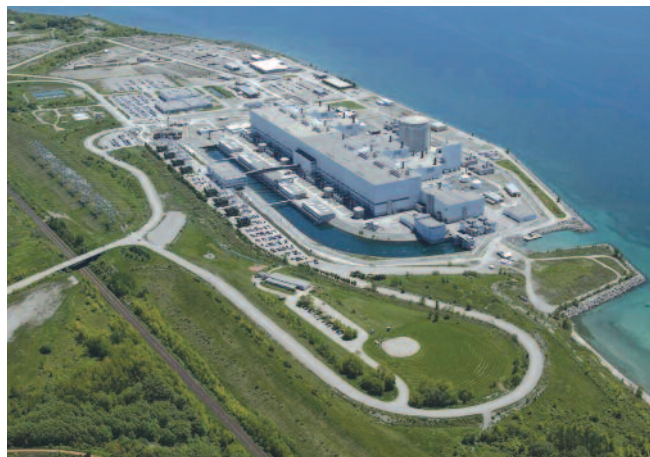
Figure 8 Four Reactor CANDU Darlington Plant, Ontario Power Generation
