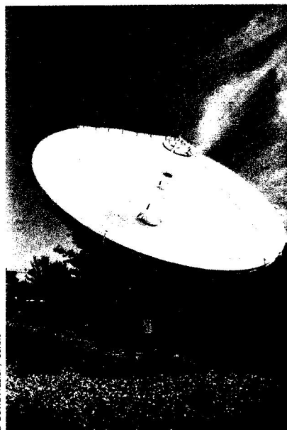
A satellite dish reflects signals to the focus of a paraboloid.
