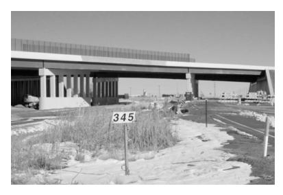
FIGURE 10. New triple-span bridge on I-70 over the transcontinental railroad near Denver's airport. The east end (right) is supported by reinforced soil. Pipeline marker is in foreground.
